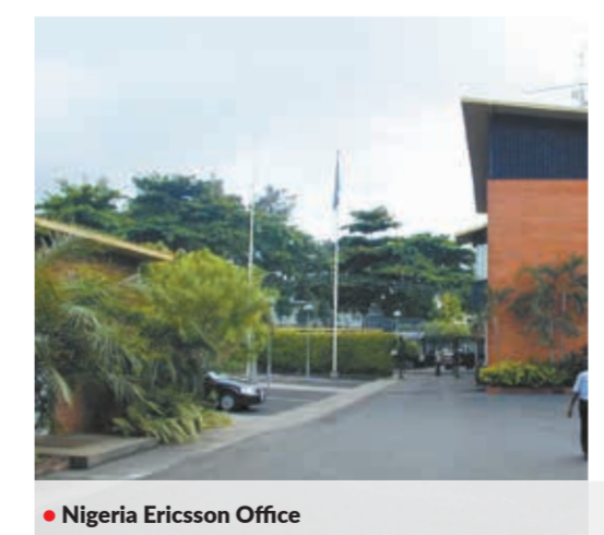
• Nigeria Ericsson Office
